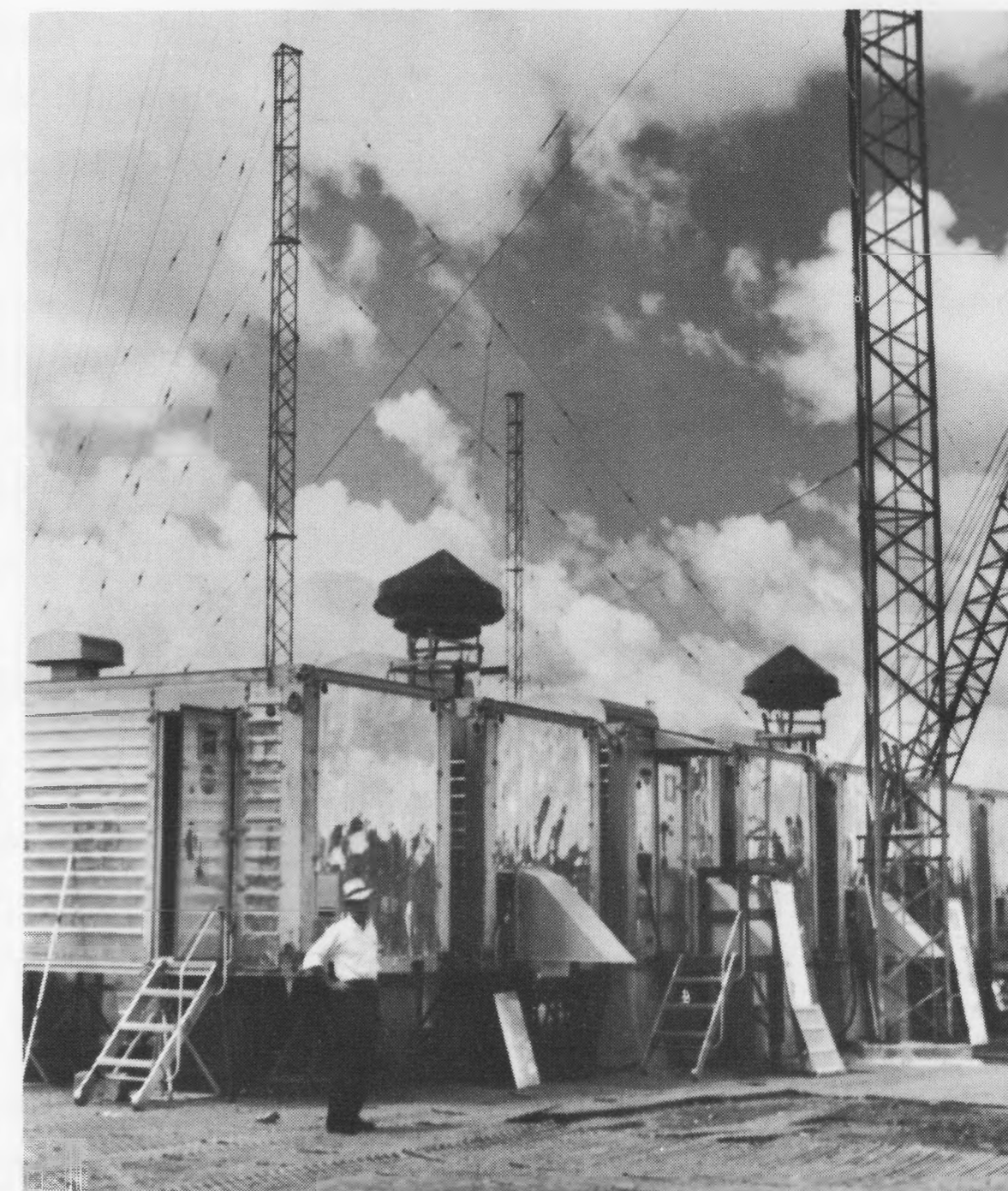
Air transportable relay station in Liberia.
